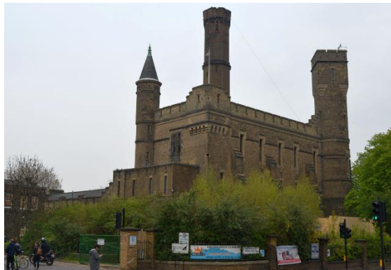
5. Green Lanes ('Castle') pumping station
