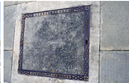
3. LCC Tramways pavement cover
