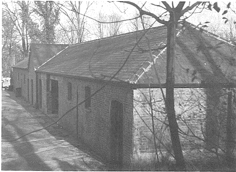
Plate 1. Former cowhouse (1883) at Cane Hill Farm, Coulsdon in 1978. The complete set of cow-stalls were in the nearer wing.
