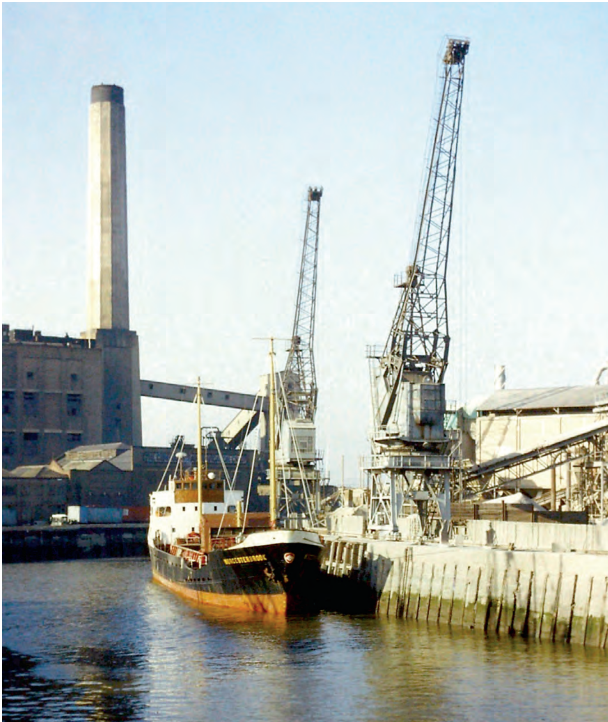
Figure 3. Looking north down Deptford Creek towards the Thames in November 1971. The power station is Deptford East HP which opened in 1953 and closed in 1983. Robert Carr
