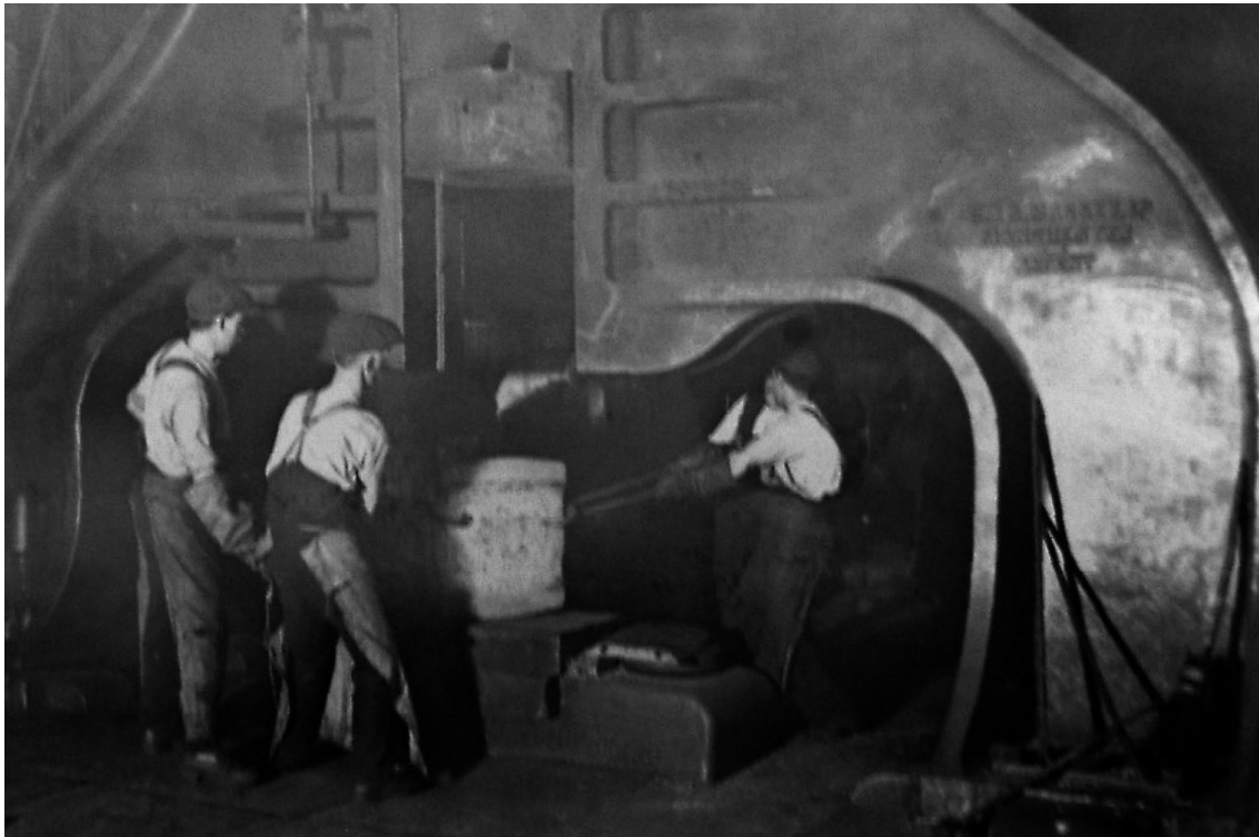
Figure 8. Stratford works 5-ton steam hammer, circa 1916
