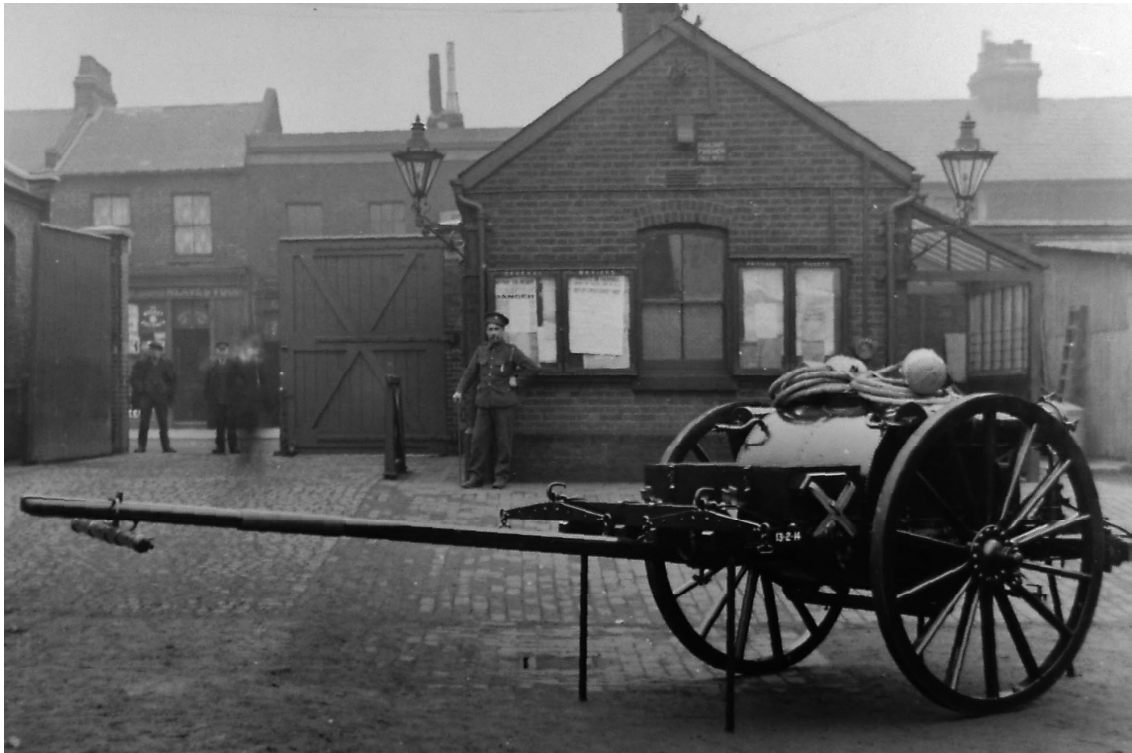
Figure 7. General Service water tank cart beside the entrance to the Stratford works, circa 1915
