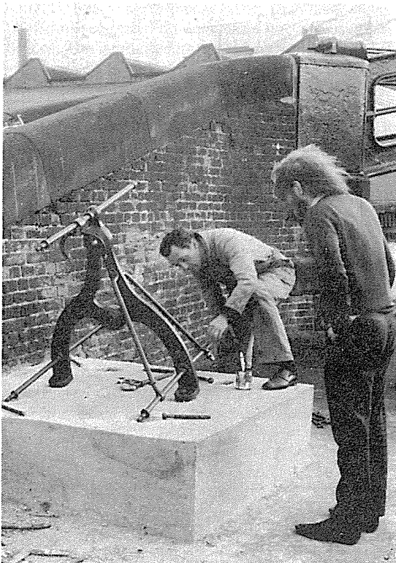
Plate 1. Paul Carter commences re-assembly of the winch in May 1972.
